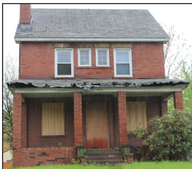
3926 Southern Blvd: DEMOLITION
