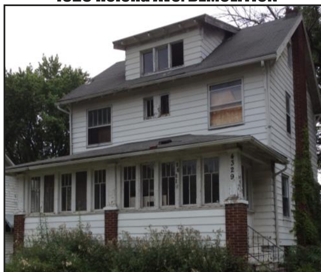
4329 Helena Ave: DEMOLITION
