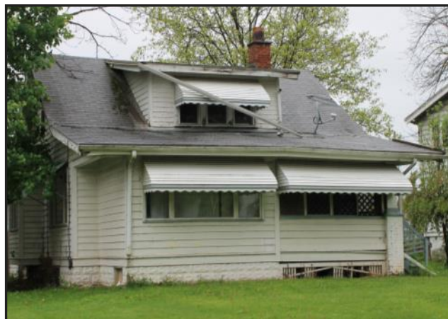
4325 Helena Ave: DEMOLITION
